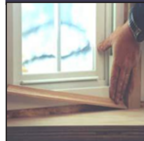
Back Seal Window Stops
