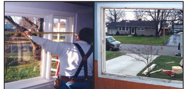
Double check all measurements prior to removing window.
