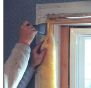
Insulate around Frame
