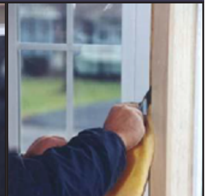
Insulate between Windows and Frame
