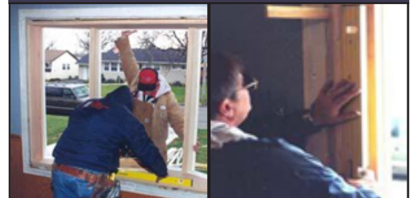
Level Bay or Bow Frame in opening
