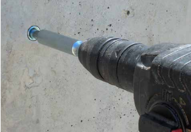
Anchor being set with SDS setting tool.
