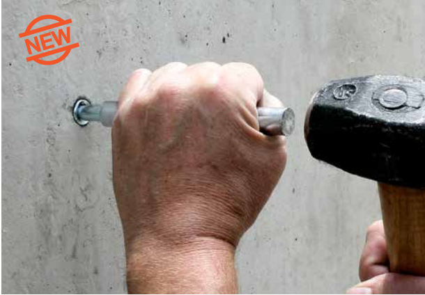
Anchor being set with hand setting tool.
